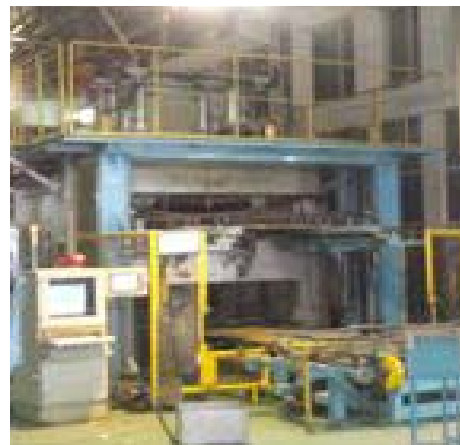
Bending furnace for bus and truck glass
